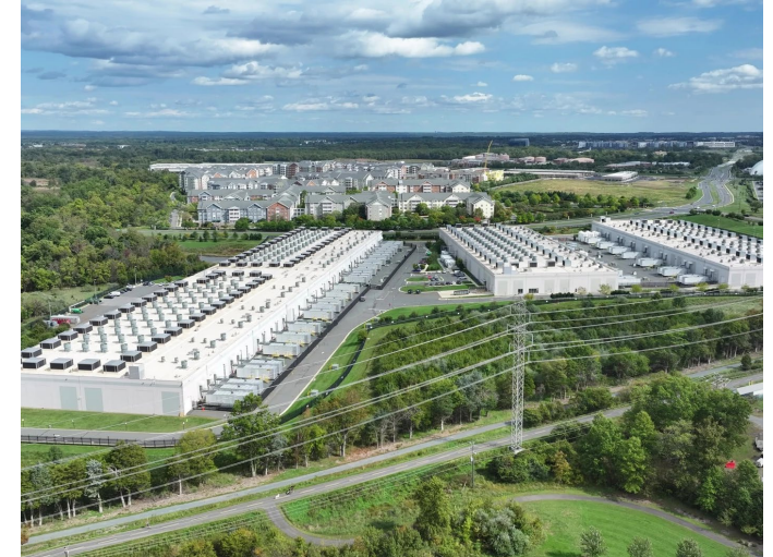
Data center (screen capture/VPN)
